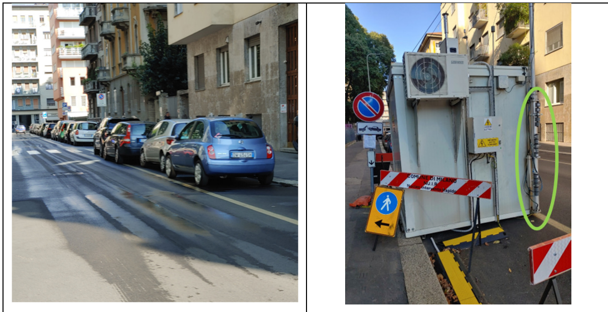
Figure 69. Intensive street cleaning in Madre Cabrini (left) and resuspension passive samplers (right).
